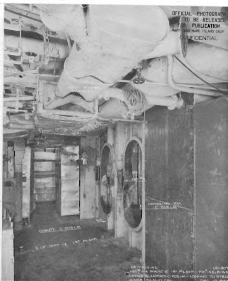
Photo 5: Hits No. 1 and No. 4 first platform crew's quarters C-203-LM looking to starboard
