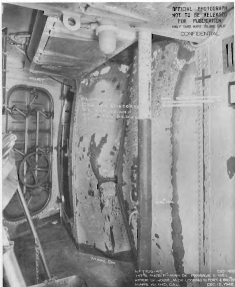
Photo 11: Hit No. 6 main deck passage C-105-L after deck house.
