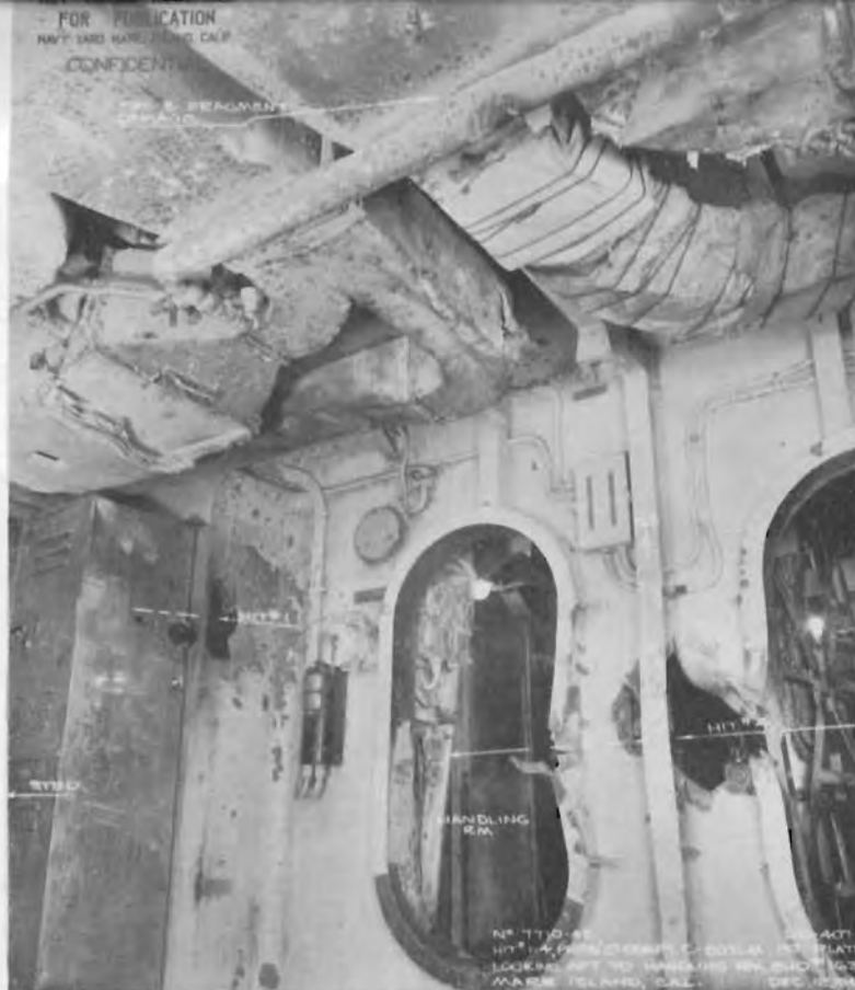
Photo 4: Hits No. 1 and No. 4 first platform crew's quarters C-203-LM looking aft to handling room bulkhead 163.
