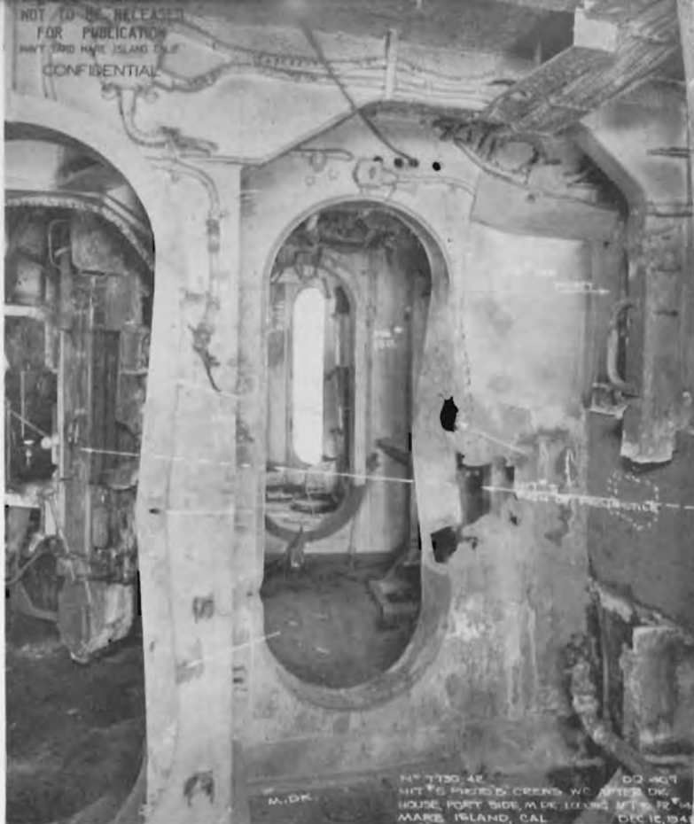
Photo 8: Hit No. 5 main deck port side after deck house looking aft to frame 148.
